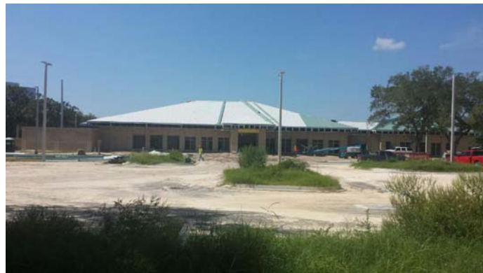
The roof is coming along!
